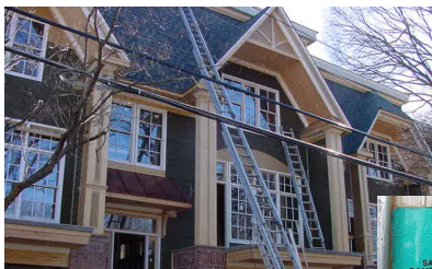
A painter was electrocuted when moving a metal ladder on this jobsite.
