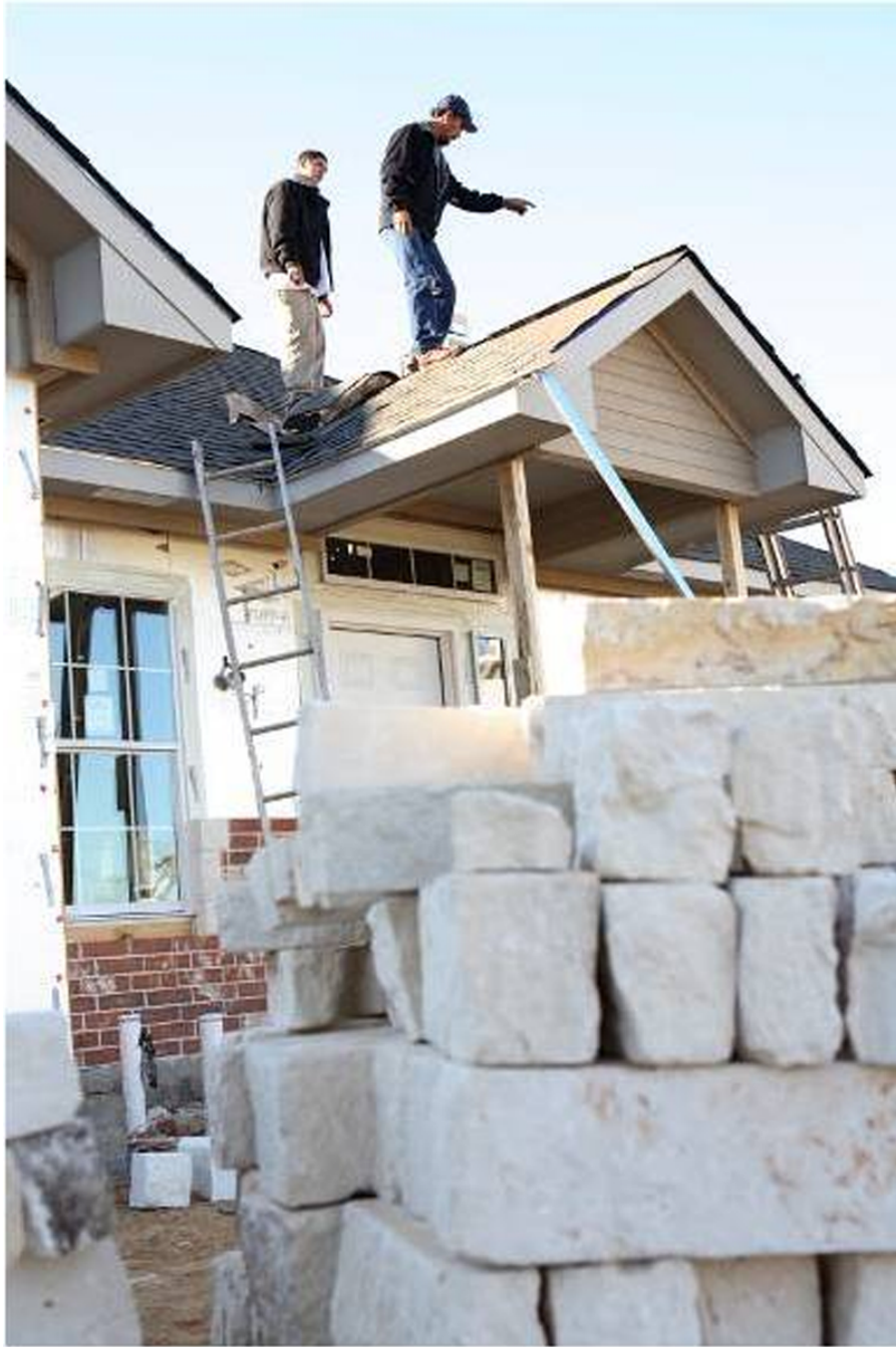
Image 889: OSHA Training Institute, Southwest Education Center http://www.elcosh.org
