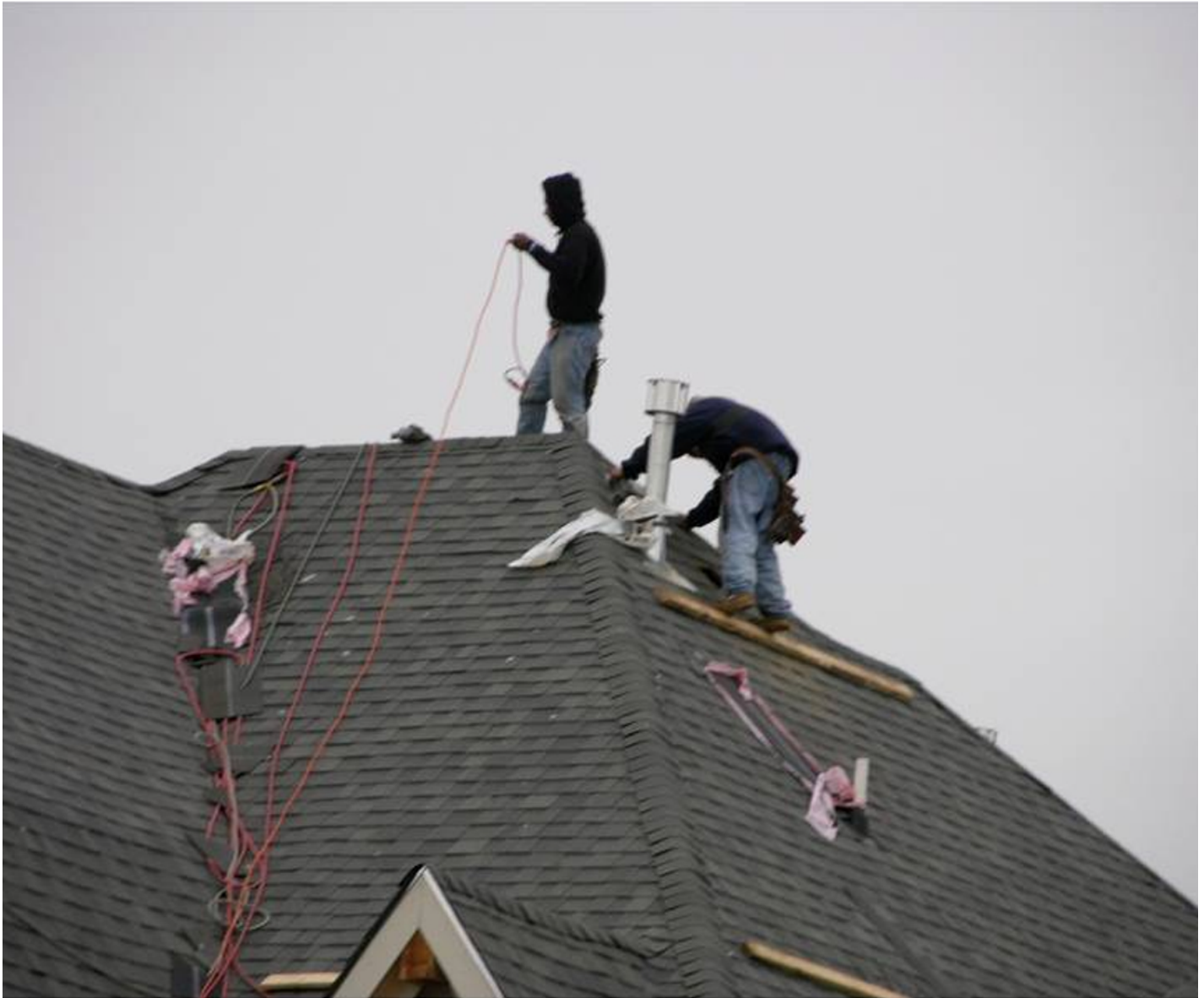
Image 821: OSHA Training Institute, Southwest Education Center http://www.elcosh.org
